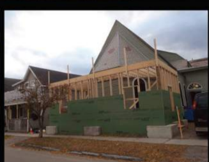
Design & Construction of a Temporary Enclosure
