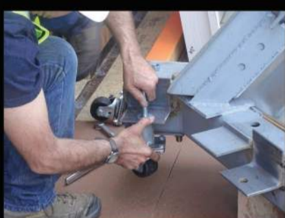
Lifted Off the Flatbed, Wheels are Installed on the Frame
