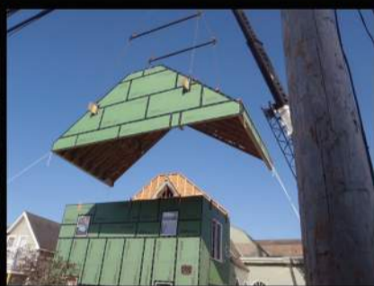
A 200ft Crane Was Used to Remove the Temporary Roof
