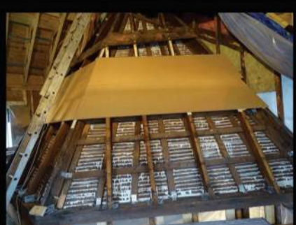
Plywood is Applied to Increase the Stiffness of the Assembly
