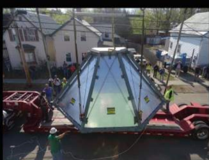
The Mural is Lowered to a Flatbed Truck for Transport
