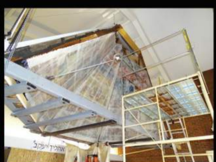
The Mural is Suspended From the Steel Frame & Suspension Rods
