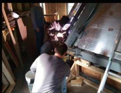
The Steel Frame is Built Around the Mural, In Place
