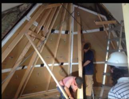
Protective Panels are Applied to the Mural Surface
