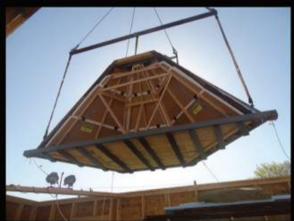
The Mural is Lifted Out of the Structure
